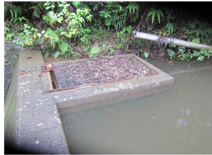
Water supply source (when rained)
