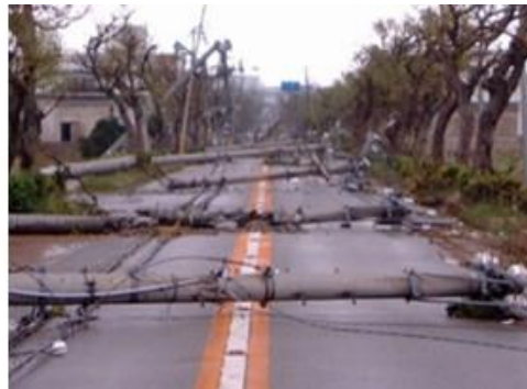
Utility poles collapsed by typhoon
