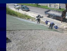
(23) Welded metal net installation
