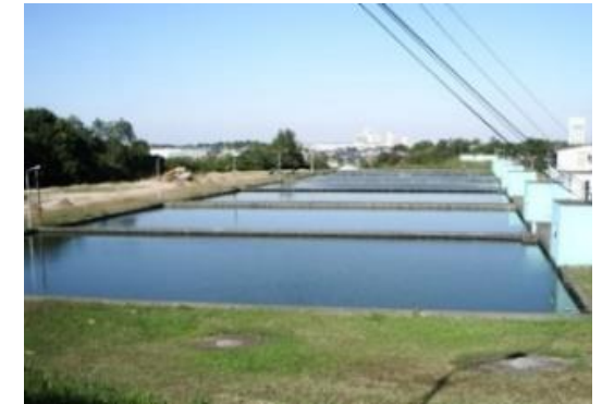
③ Water supply, water purification
