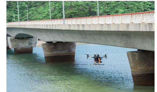
Bridge inspections using drones
