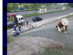
(22) Sheet installation (SP type)
